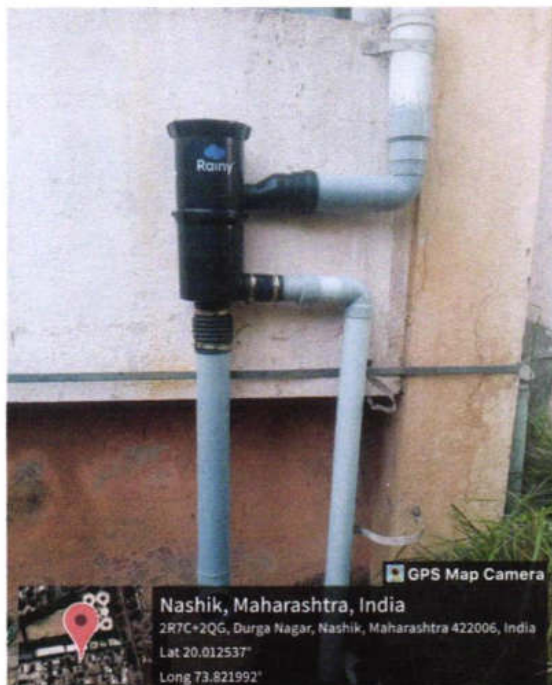
Fig. 5.: Rain Water Harvesting System
